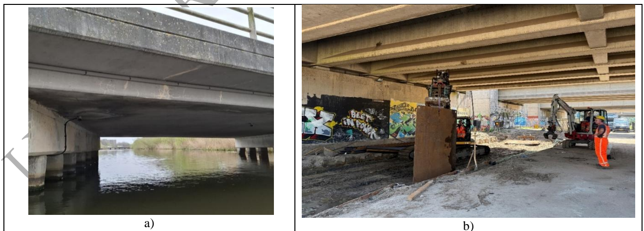
Fig 3. Photos of (a) a reinforced concrete slab bridge and (b) a prestressed concrete girder bridge.
